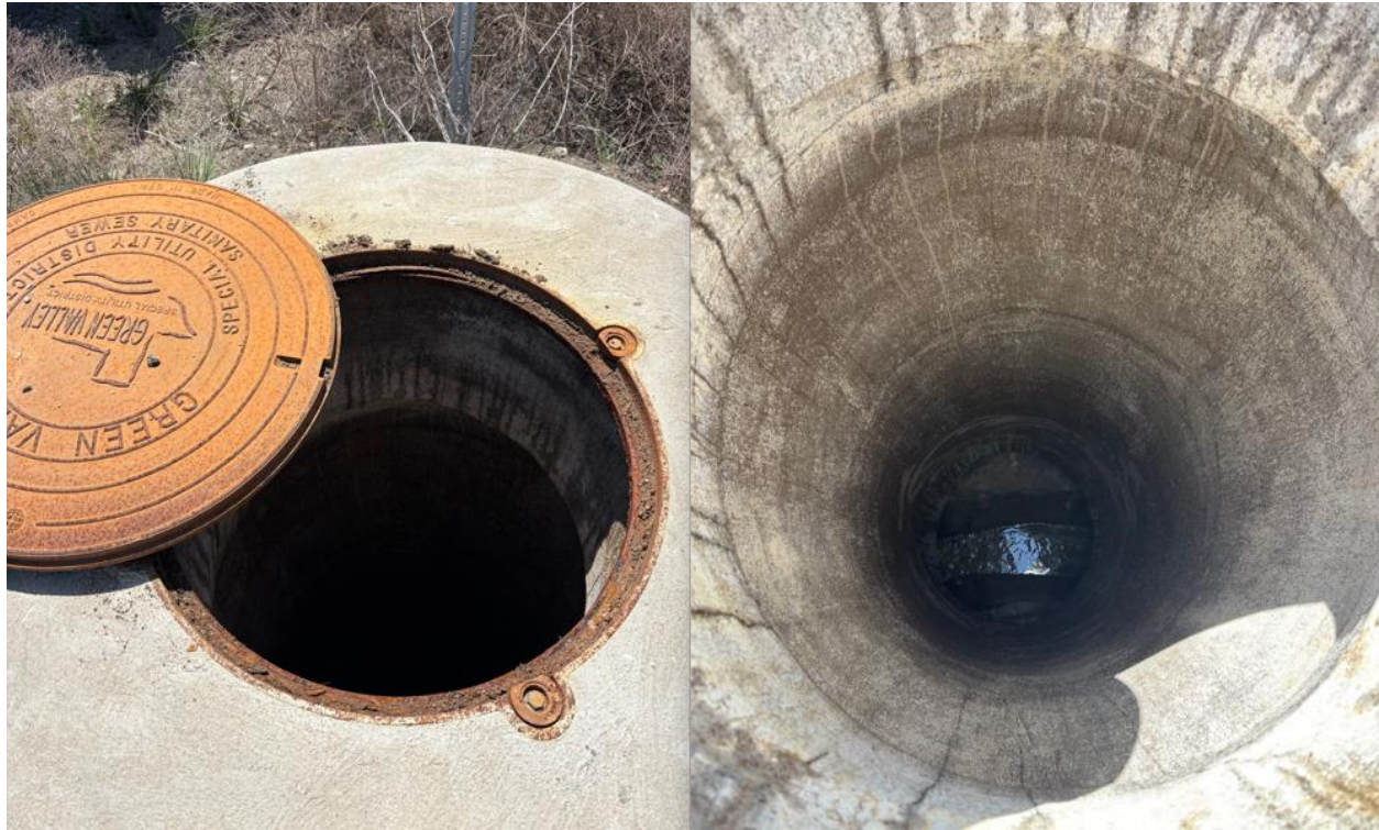
Figure 4-6: Wastewater Manhole - MH-SC-0074
