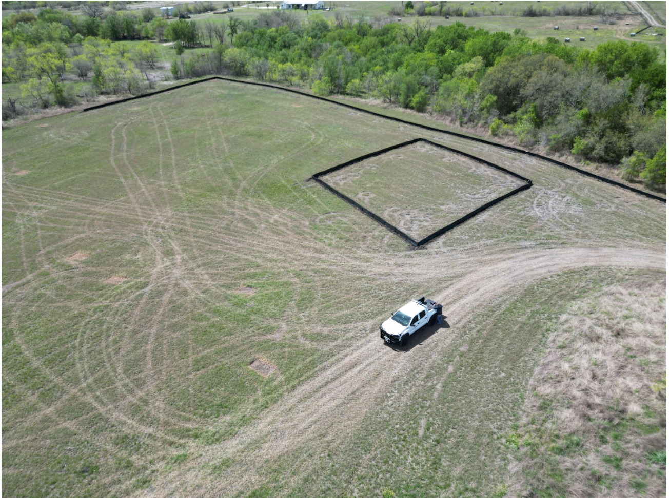
Clearwater Creek WWTP Lift Station Site
