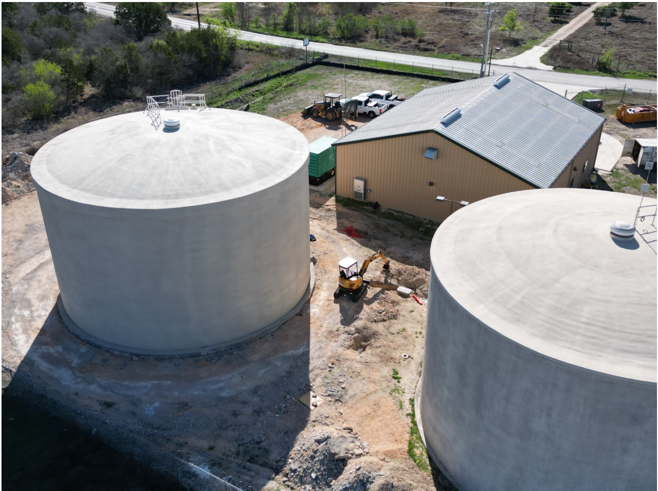
The new 0.5 MGD Ground Storage Tank at Plant 11
